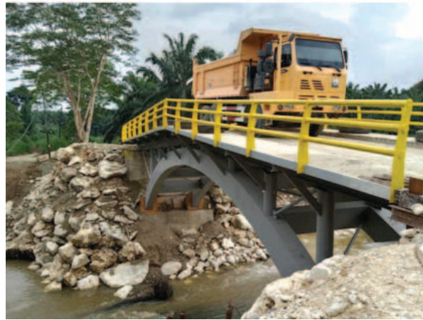
Heavy truck crossing through the Newly Constructed Taliwas Bridge
