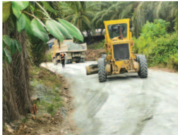
Road maintenance and upgrade of road Jalan Taliwas
