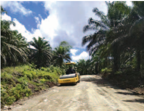
Road Upgrade and maintenance at Jalan Silam - Ulu Segama in progress
