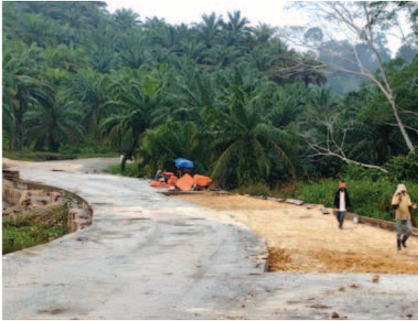
Construction Work at Sg. Upak River crossing
